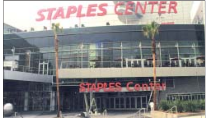
Installation by Giroux Glass, Los Angeles, CA.
