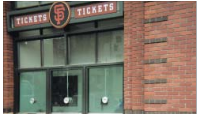
Installation by Architectural Glass & Aluminum, Oakland, CA.
