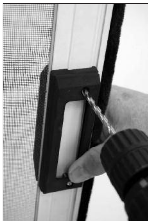
Diagram 11 - Attaching Pull Handle
