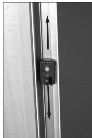
Diagram 12 - Adjusting Plastic Hook Latch
