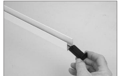
Diagram 6 - Installing Plastic Angle Brackets
