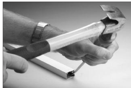
Diagram 8 - Crimping Weatherstrip Channel
