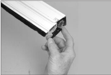
Diagram 4 - Installing Pull Bar Guides
