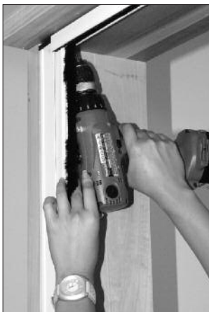
Diagram 10 - Attaching Top into Header
